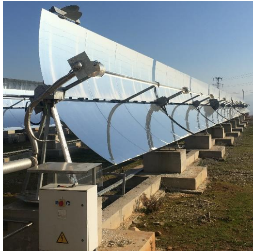
Figure 3.2. Silvered mirror reflectors of PTSC at ADU Solar Field
