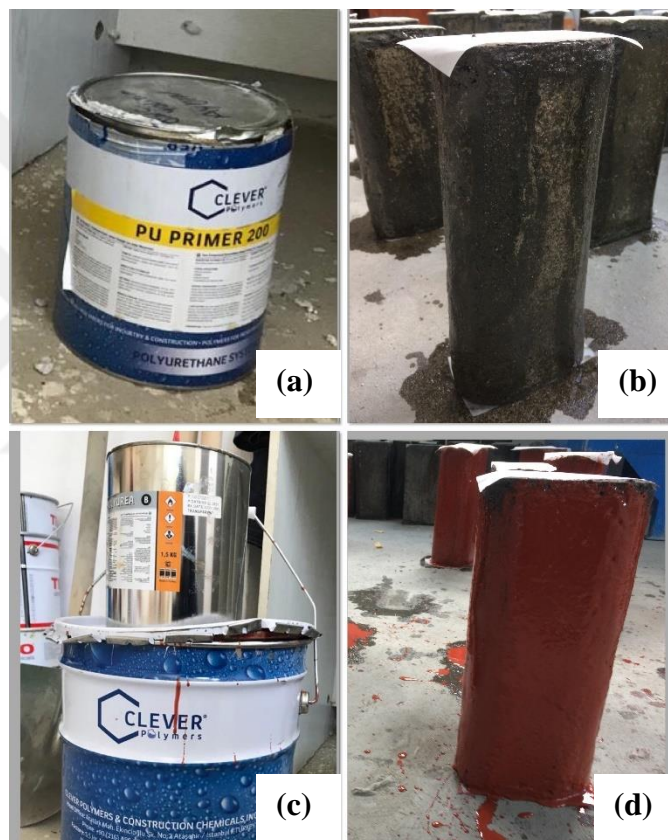
Picture 3.7. (a) The polyurea primer, (b) the polyurea primer application, (c) the components of the polyurea and (d) polyurea application
