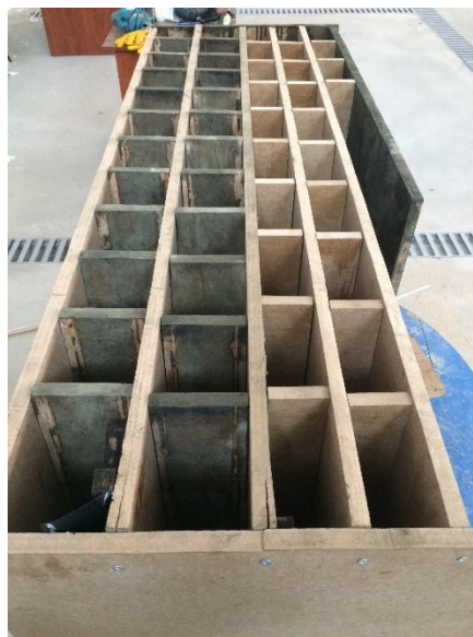
Picture 3.1. The formwork
