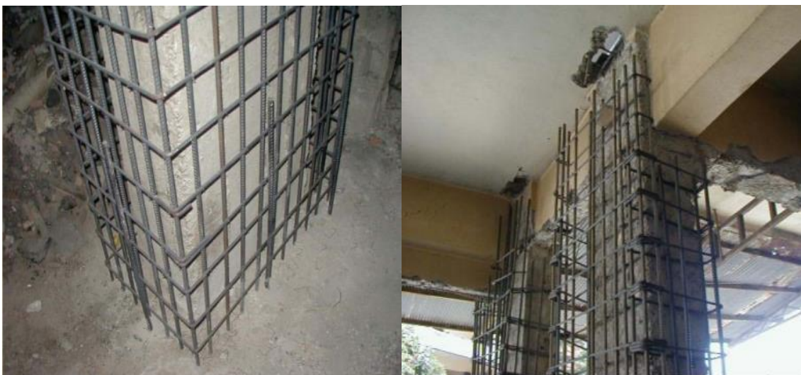
Picture 1.1. The column confined by a new reinforced concrete layer (Altin, 2008)
