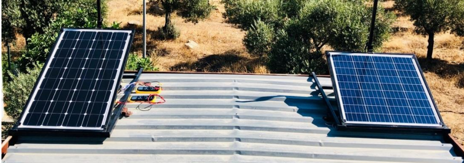
Figure 3.7. Monocrystalline and polycrystalline photovoltaic solar panels
